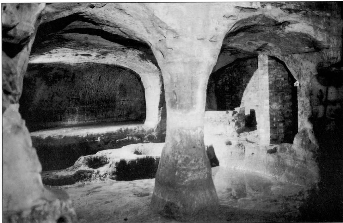
Pillar Cave in the Drury Hill caves system. A flared pillar supports an unusually wide roof; brickwork has been added to the cave, in the background, but the site is now preserved beneath the Broad Marsh Centre.
