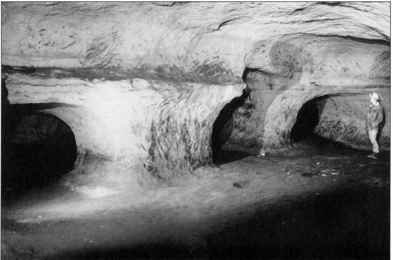
One of the larger galleries in Rouse's sand mine west of Mansfield Road; the pillar-and-stall plan and the two levels of working are visible.
